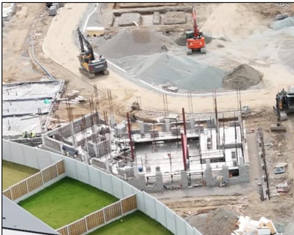
Figure 2 Construction Progress on Creche Building
